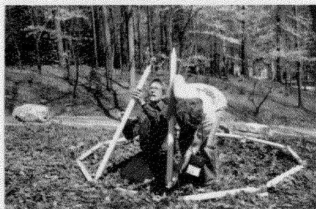
Work begins (left) on constructing a hyperbolic paraboloid
