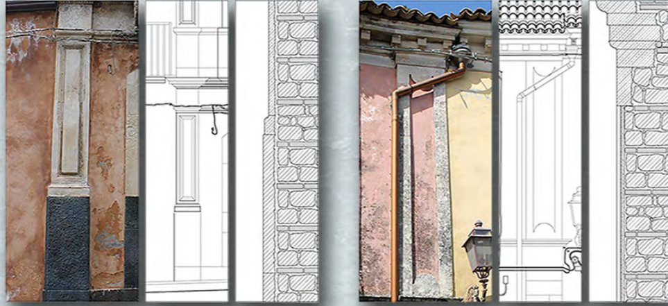
Lesene (Pilaster Strips)
