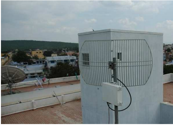
Figure 6: The Theni to Vijerani link in the Aravind network was completely obstructed by a newly constructed elevator shaft. This problem was not resolved until we visited Theni after 2 months.
